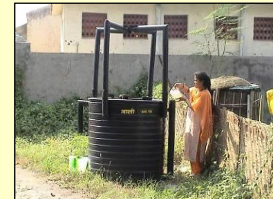
ARTI home biogas system (India)
